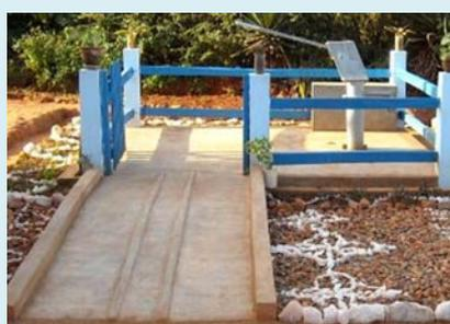
In the accessibility audit, Andry found reaching the water point was a challenge as the ramp was too steep and the gates opened outwards (left photo). The water facility was rehabilitated so that the gates open inwards, the ramp was widened and the gradient made less steep. Wheel guidance was introduced on the ramp and the edges were raised to assist wheelchair users and visually impaired people (right photo).
