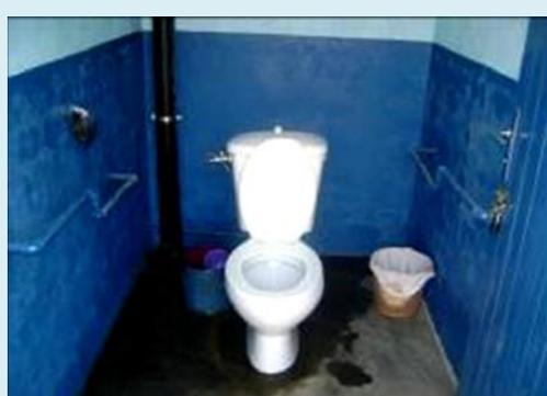
This school toilet was modified to include a toilet seat and hand rails to enable greater access (left photo). However, the cubicle was too narrow to allow a wheelchair user to turn; this meant Andry had to turn herself around using the rails for support. The support rails were also too high. The re-modelled version is 1.5 metres wide which allows Andry to turn in her wheelchair inside the cubicle. The lower rails allow a person to transfer themselves using one rail (right photo).
