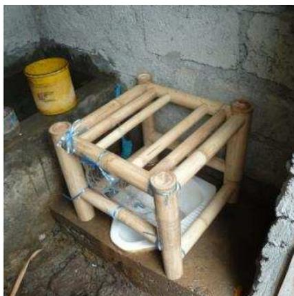
A simple bamboo frame with splash guard made of plastic bottles
